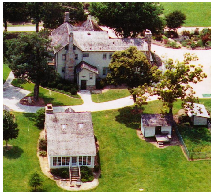
Cabin and Federal era house at Bennett Bunn Plantation along with its farmland is on the National Register as an individual listing.
